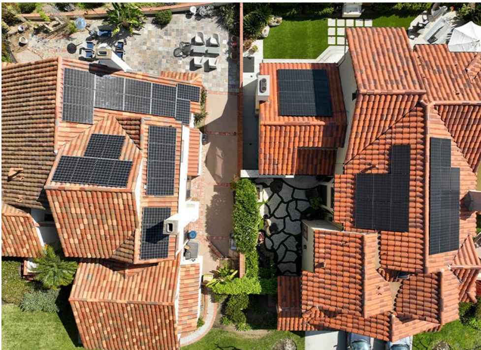
California has 1.5 million rooftop solar arrays generating 12 GW of electricity, the CPUC said. | Shutterstock
