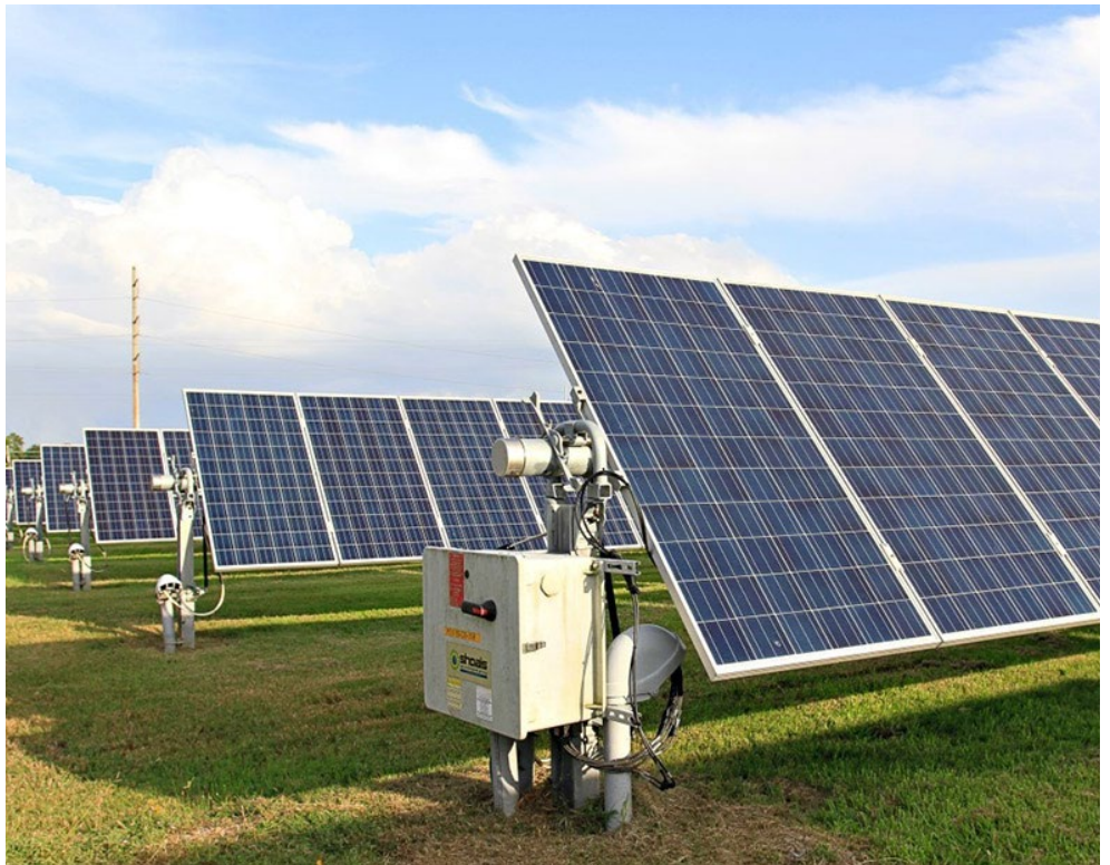
Entergy solar generation in New Orleans | Entergy
