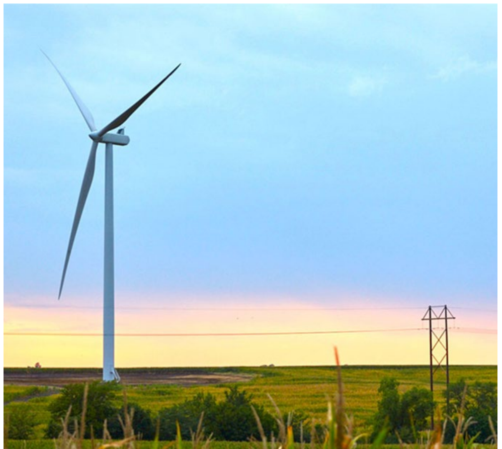
The Clear Creek Wind Project | Mortensen Wind Energy Group
