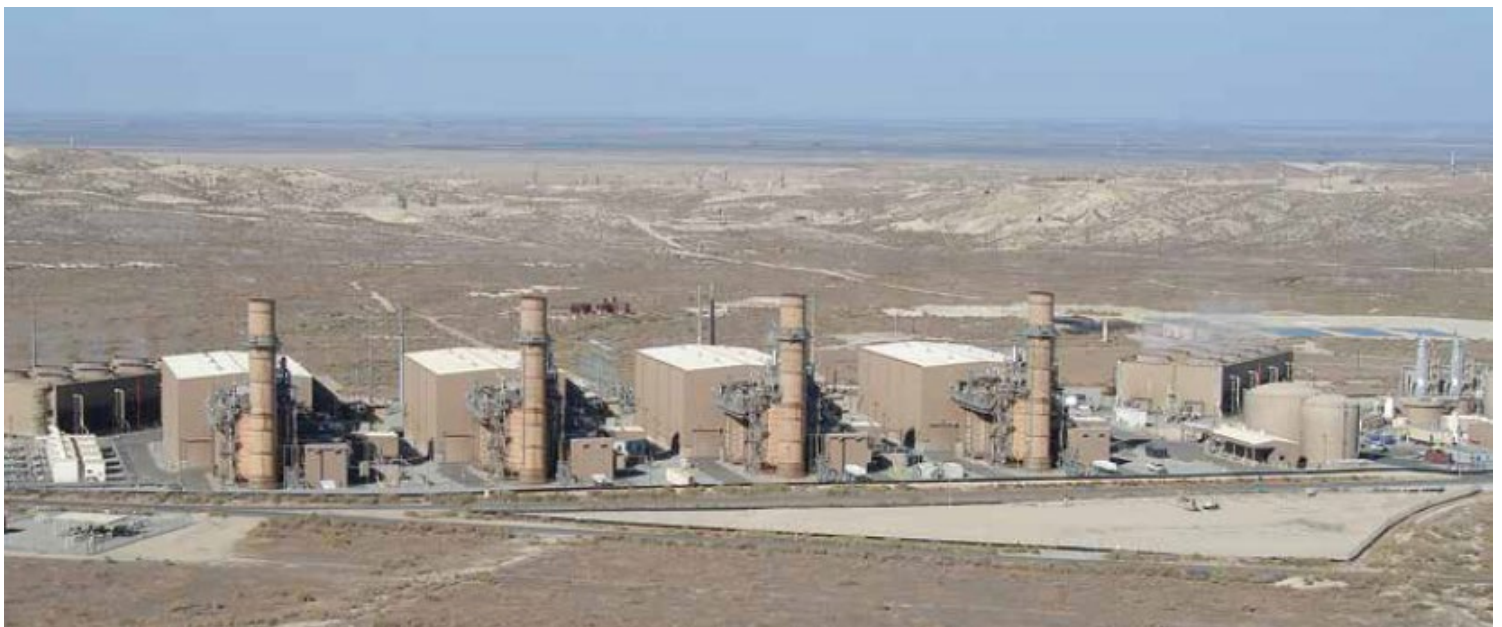
La Paloma Generating Plant in Kern County, Calif. | MeeFog
