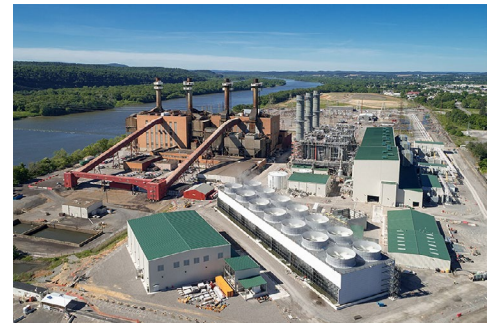
Panda Hummel Station, a 1,096.5-MW combined cycle plant on the Susquehanna River near Sunbury, Pa. | Bechtel Corp.
