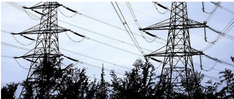
| Central Main Power
