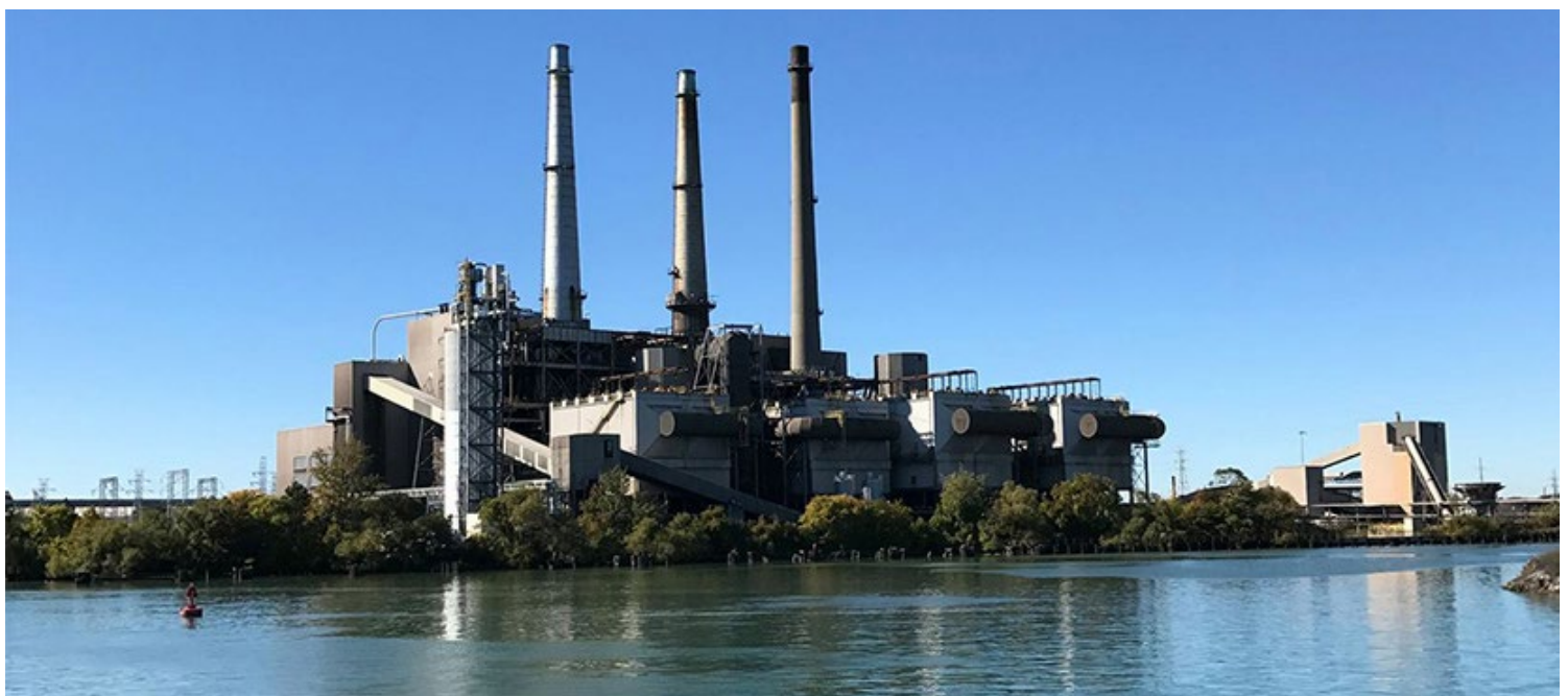
DTE Energy closed its 358-MW River Rouge coal-fired plant near Detroit at the end of May | Bridgepointe
